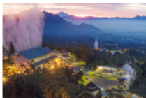
Image credit: Star Energy Geothermal
